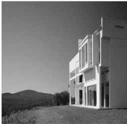
Fig.1: Eisenman House 1967 Peter Eisenman
